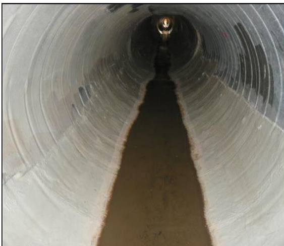
Figure 2: Hand-laid MIR-940 and spray application of MIR 950
