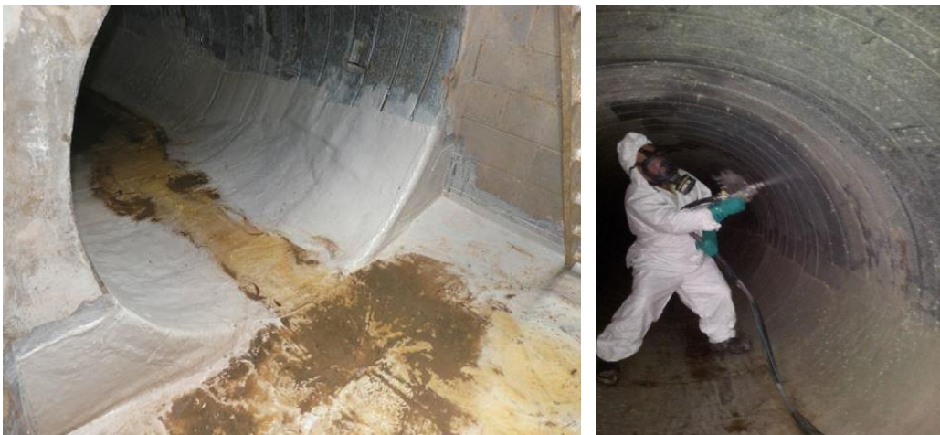
Figure 2: Hand-laid MIR-940 and spray application of MIR 950
